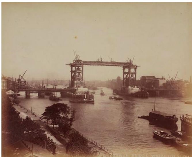
TOWER BRIDGE UNDER CONSTRUCTION IN 1892
