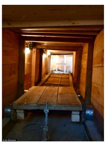
Tunnel vision: A tunnel reconstruction showing the trolley system.
